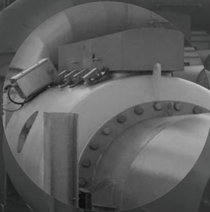
Isolation of a pipe with EXKOP® QV III.
